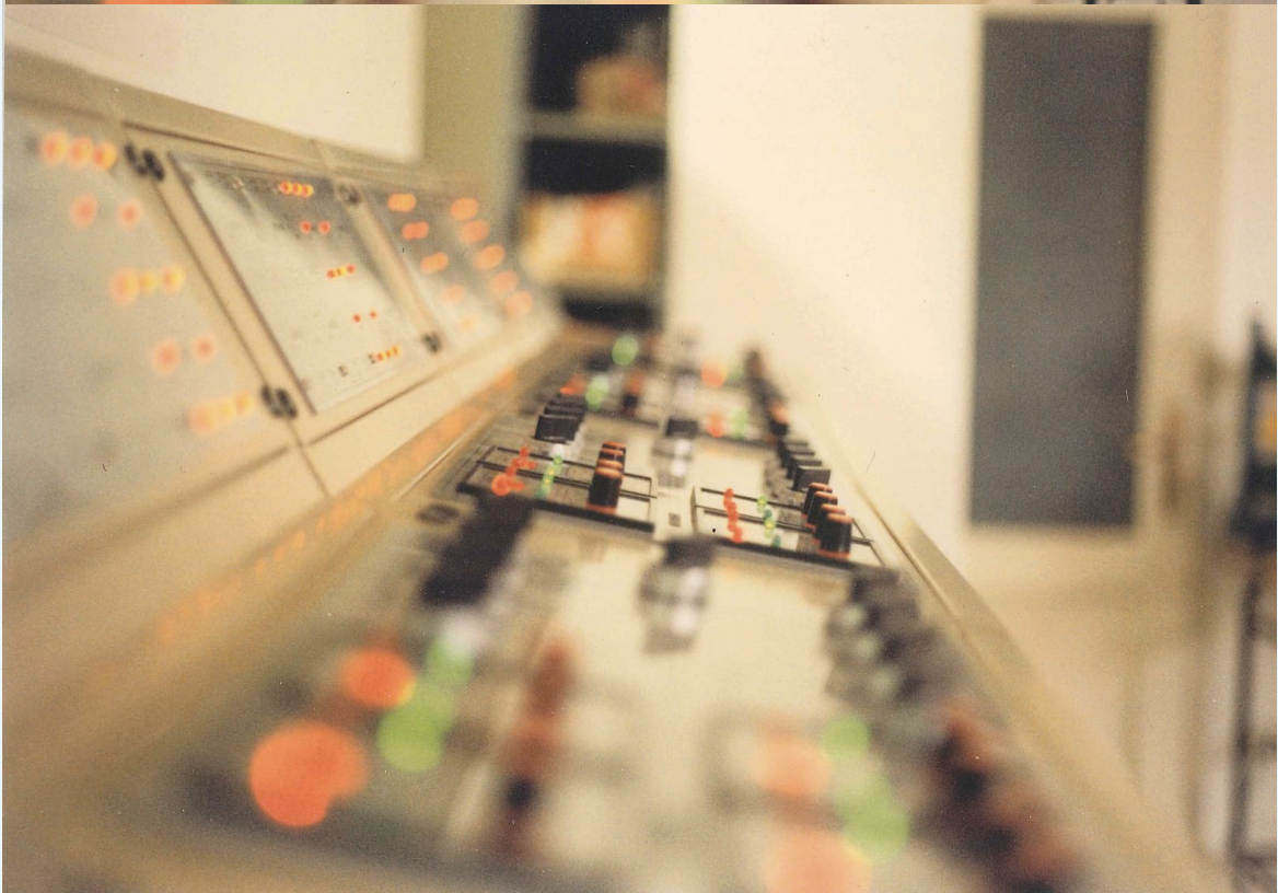
Greenhouse controls in Saudi Arabia Controllo serre in Arabia Saudita
